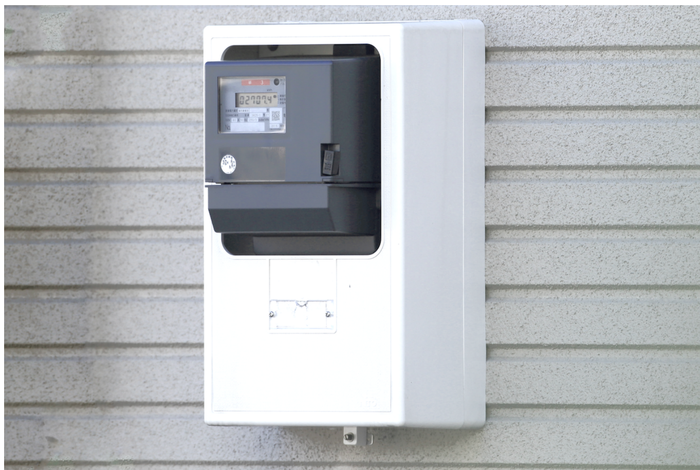
Figure 1. Example of a smart meter commonly used in Japan to collect household electricity consumption data. This figure shows a typical smart meter, usually installed outside Japanese residences. In this study, 30-minute interval electricity consumption data in watt-hours were obtained through these meters using a home energy management system, a home gateway, and the wireless smart utility network. This image is for illustrative purposes only and does not depict the actual device used in the study.
